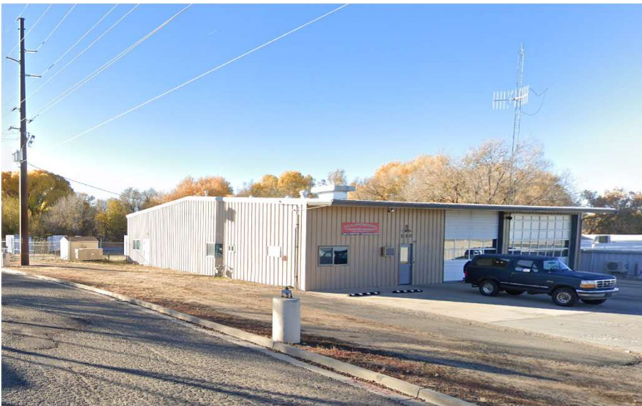
Existing Station 72 · 530 6th Street
